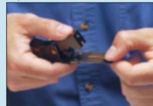
Step 2: Cleave the fibre
