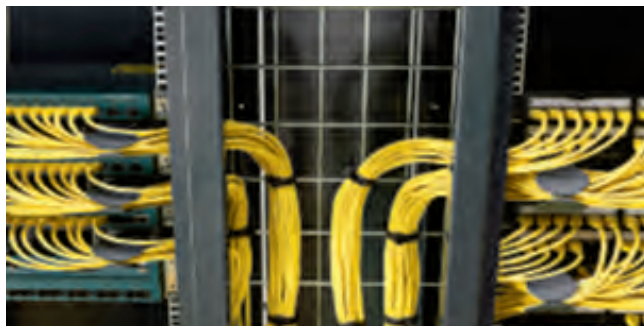
Dedicated space for cable management with easy access via door to cabling unit
